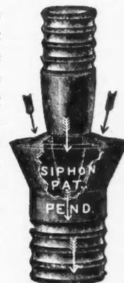
This is the Device Thru Which the Water Is Forced by Water Pressure from the Tub Into the Sink.
