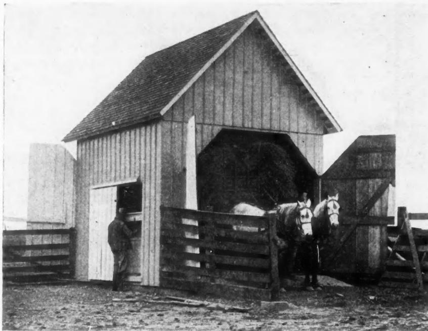
Well Built House for Farm Platform Scale. Every Farmer Should Have a Scale and Should Protect It from the Weather by Means of a Suitable Building. The Doors Enclosing the Platform, and the Fencing Leading up on Each Side, Make It Easy to Weigh Live Stock Either Singly or in Flocks.
