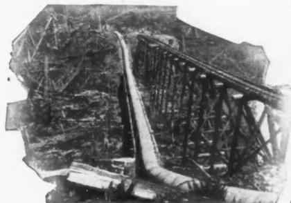
28-Mile Reinforced Concrete Pipe Line, Sooke Lake Aqueduct, Victoria, B. C.
