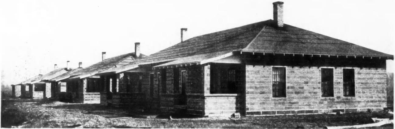
Row of Double Houses at Brazil, Ind., for the Employees of the Clay Products Company. Using Their Own Material—and It Is a Logical One of the Construction of Workingmen's Homes—these Houses are of Tile Construction.
