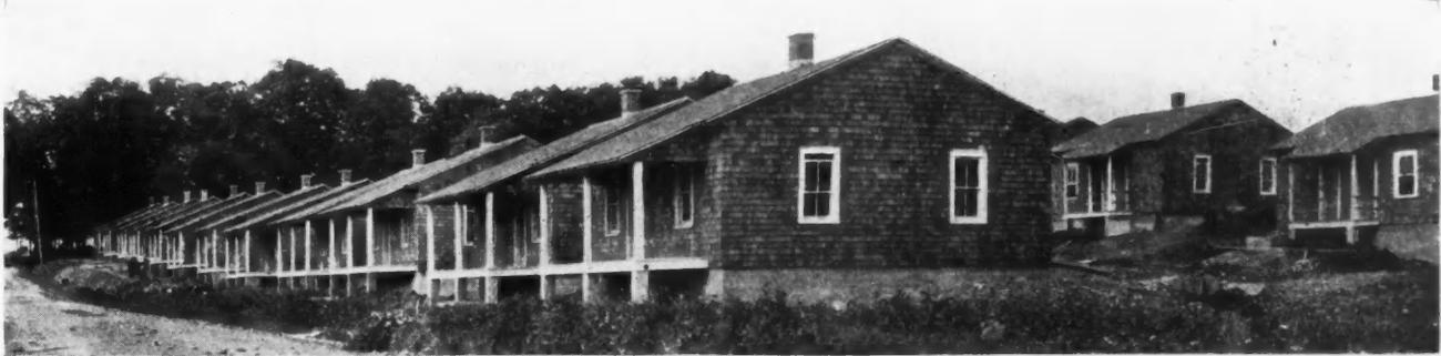
Group of Four-Room, Shingled Cottages Built at Milltown, N. J., for the Michelin Tire Company. Fifty-Three Houses Were Built Complete in 56 Working Days, by the John W. Ferguson Company, at \$1,125 Each.
