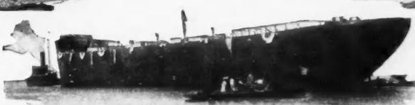
7900-Ton Reinforced Concrete Cargo Steamship Faith, Largest Concrete Vessel Afloat
