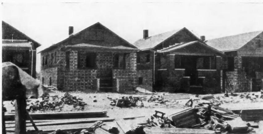
Four-Room Cottages of Tile Construction at Gary, Ind., Erected by W. L. Plew & Company. The Same Floor Plan as Shown on the Left is Used for All. Variety of Exterior is Gained by Having One Stuccoed, Another Faced with Brick, and a Third of Matt-Face Tile, etc.
