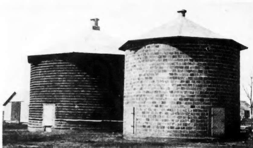
Ten Thousand-Bushel Round Corn Crib and 8,000-bushel grain tank, both of hollow clay tile on the farm of R. C. Head, near Jefferson, Iowa.
