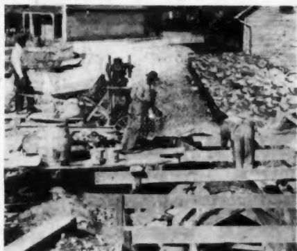
Half Bag Archer Mixer Delivering Direct Into Forms on Sewer Conduit Work
