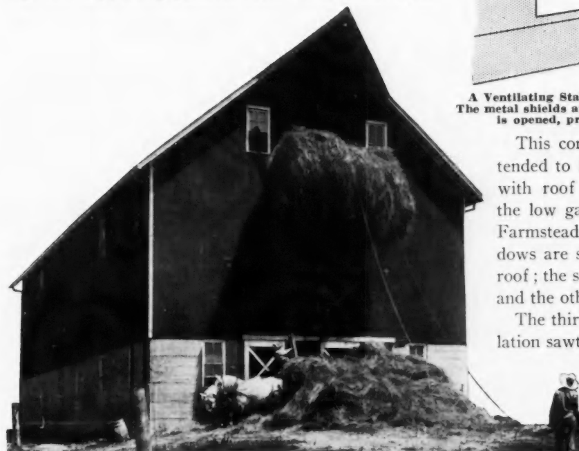
Getting in the Hay at the Oakland Farm, Wayne, Ill. Modern hay carriers hoist immense loads. Hay doors in the ends of the barns are preferred by most farmers today; they find that barns arranged to drive in with the hay are too expensive.
