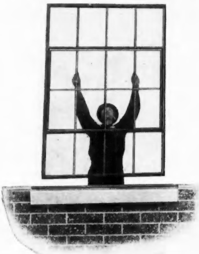
One Man Can Lift a Steel Sash Unit and Set it in Place on the Sill.
