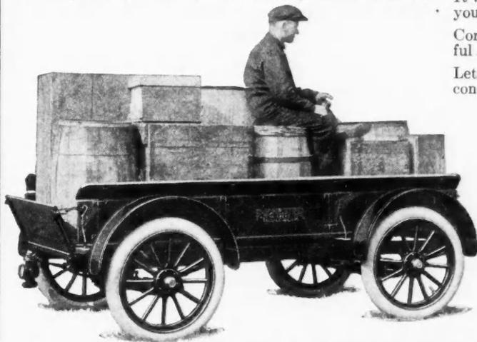
It is built exceptionally low, making it easy to load and unload, and can be drawn over the country road at a speed of 25 miles an hour safely and without skidding or jostling.
