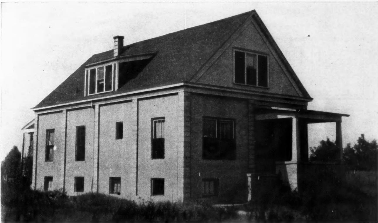
Residence Built by Using New System of Block Pilasters and Poured Curtain Wall Panels. A very pleasing architectural effect is produced.
