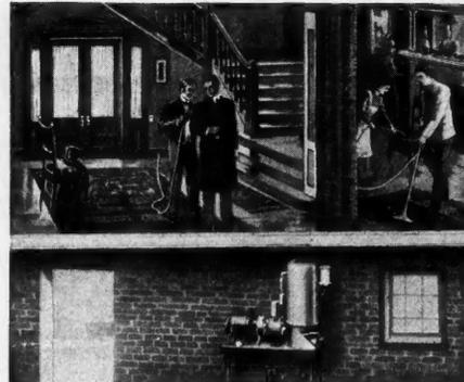
Thurman No. 2 Electric-Driven Stationary Vacuum Cleaner Installed in Basement of a Residence.
