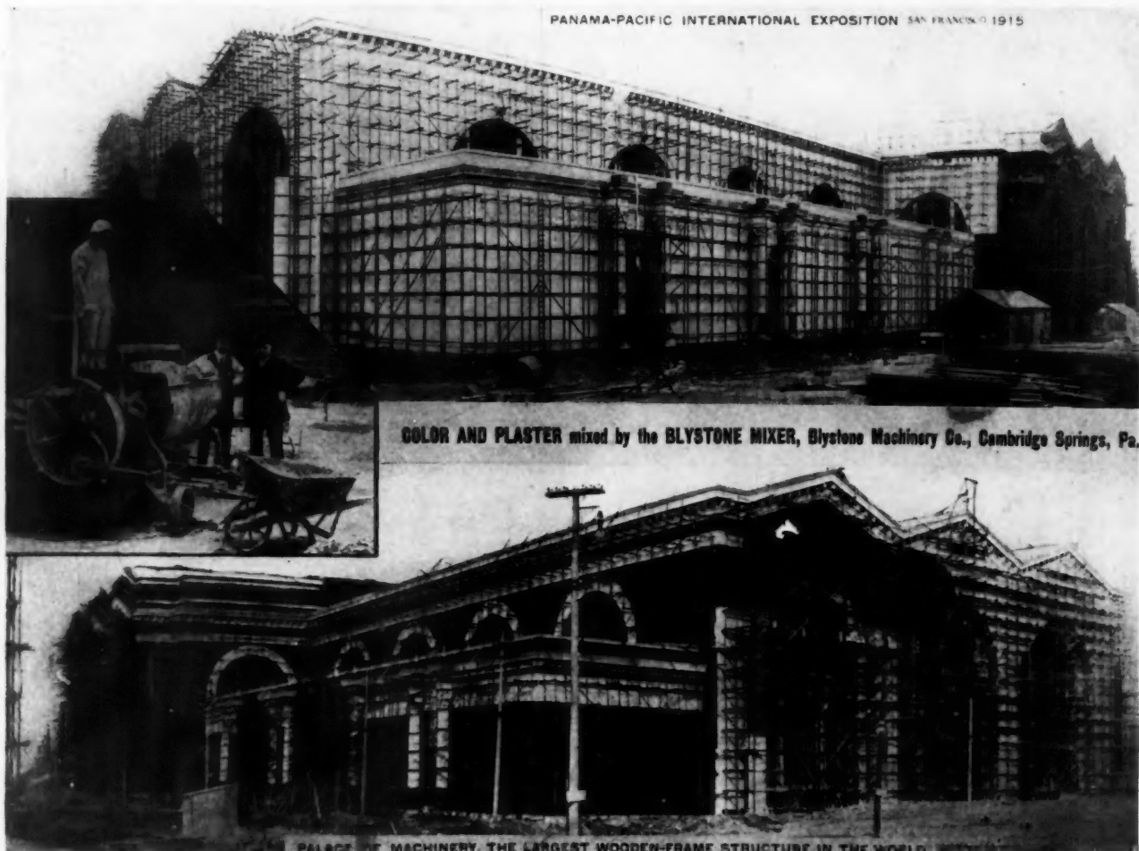
E. T. Thornton (in the Black Coat) and His Blystone Batch Mixer which Mixed all the Plaster for this Huge Fair Building
