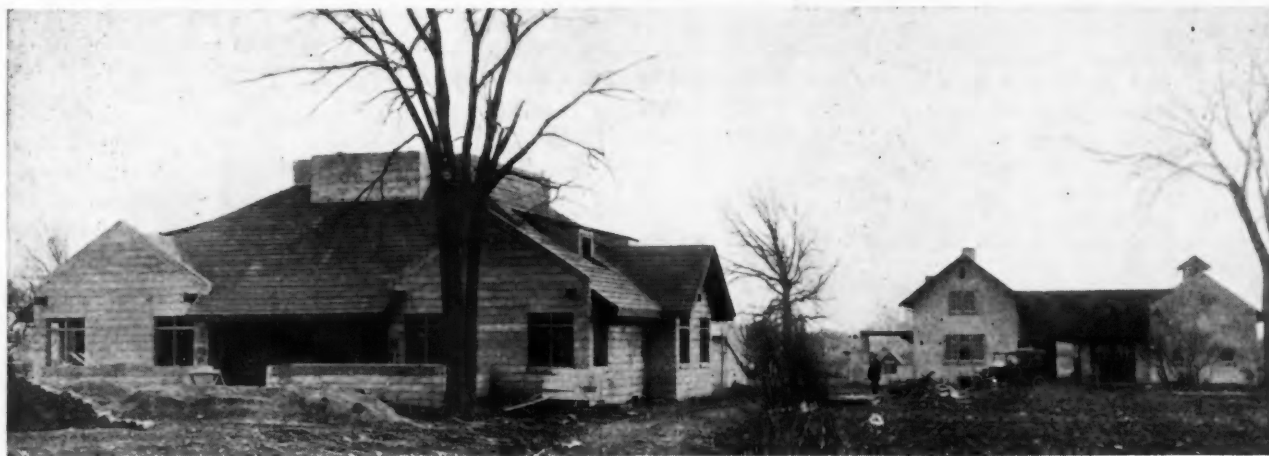
Residence Country-Place Structures of Dr. Charles R. Pullen, Rochester, N. Y., Built with Double Concrete Walls Cottage, Garage, Stable
