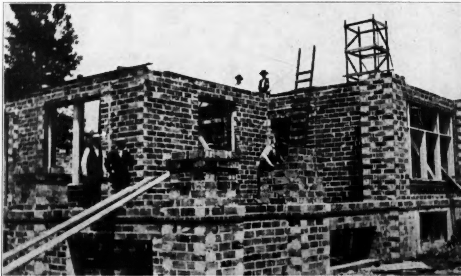
Laying up Davenport Vitrified Building Blocks, to Be Finished Later with Stucco
