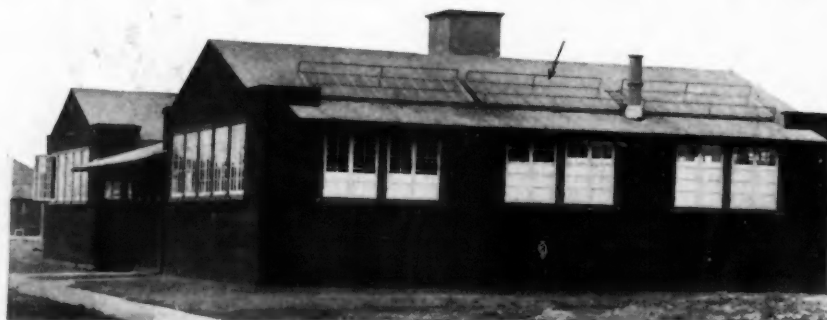
A Park Playground in Los Angeles. Solar Heaters on Roof Warm Water for Shower Baths
