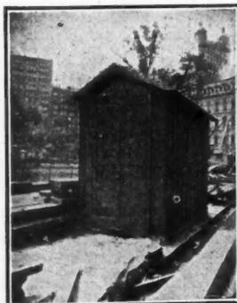
**Prudential Steel Buildings** are also Portable. We make them in **Telescoping Unit Sections** of No. 22 and No. 24 Galvanized Steel, either of single or double walls.
