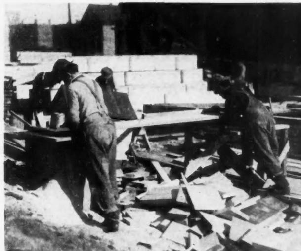
Portable Saw Rig Sawing Form Lumber on Big Reinforced Concrete Job for the Hanson Construction Co., Milwaukee, Wis.
