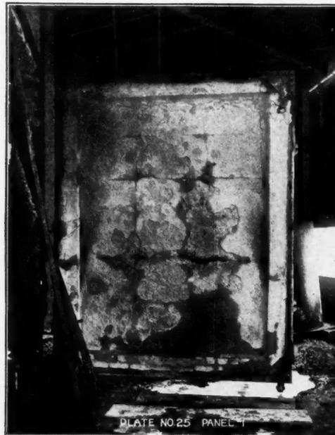
Photo of 5½" Partition—Cement Plaster on Metal Lath, 2x4 Pine Studs—After Two Hours Firing at 1912° Maximum Heat
