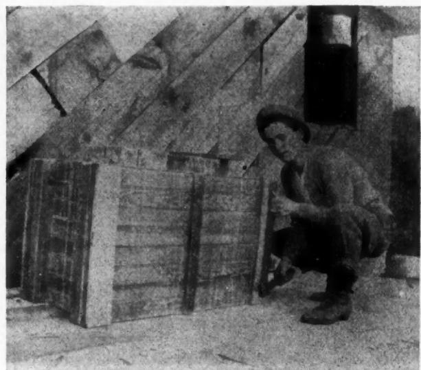
Tightening up Forms Before Filling With Concrete for new Section of Chimney
