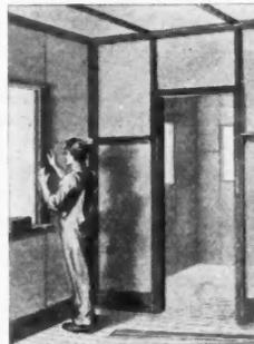
Before putting on decorative strips center nails are counter-sunk, sizing or first coat of plaster depressions filled and panels painted.
