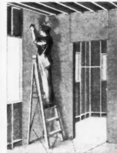
Nailing up panels, using flat-head nails  $\frac{3}{4}$ " from edges, 3" apart and bungs-head nails 6" apart for centers.
