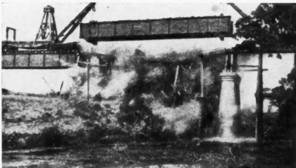
Fig. 2. Dynamiting the Old Trestle to Make Way for the Girder
