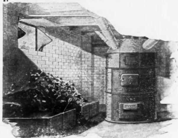
Notice the plate at the top of the frame? That covers the glass when the chute is open. It swings at the outer end and drops down, forming the bottom of the chute.
