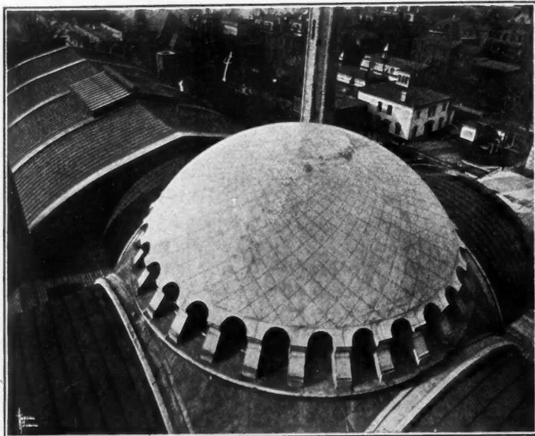
Tin Roofing for Curved Surfaces—Square Sheets Laid Diamond Shape
