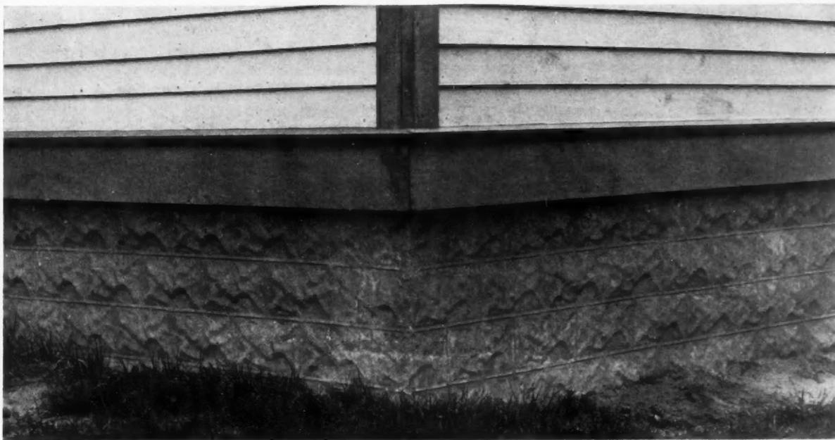
Poured Concrete Foundation Made to Resemble Blocks by Use of Rock-Faced Sheet Metal
