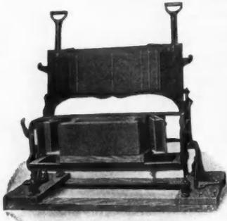
**"The Miles" No. 5, Down Face, Wet Concrete Block Machine**
