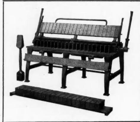
Is the fastest Hand Brick Machine on the Market; will make plain, veneered and ornamental face and shape; all perfect, smooth brick, true to size and design. Send for catalogue giving complete line of Mixers and Brick Machines.
