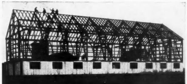
when last rafter was being put up and the basement siding on. There are sixteen double windows and six single windows in the barn. The work was started Oct. 29, 1907, and in nine and one-half working days of nine hours each, with eight men working, the barn was as shown in photo. W. S. Ford, of Burton Ohio, was the contractor.
