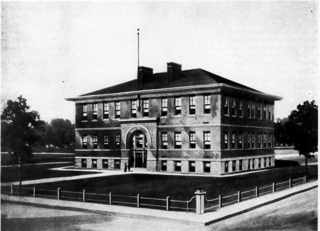
been done in a most admirable manner by G. W. Ashby in planning the eight-room school building shown herewith. Its location is in a southern state where the heating question is not a serious one. The expensive basement furnace system has accordingly been omitted. This has made possible a very
