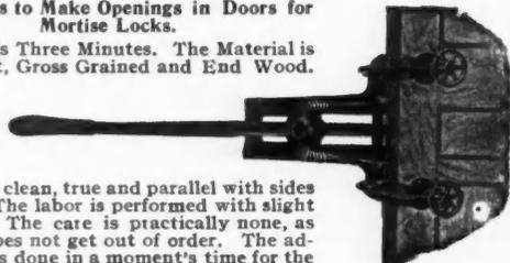
The job is clean, true and parallel with sides of door. The labor is performed with slight exertion. The care is practically none, as the tool does not get out of order. The adjustment is done in a moment's time for the different sizes. The cutters are five in number and cover locks from 1/2 inch to 1 1/2 inches thick. Thin doors are handled as easily as thick doors.
