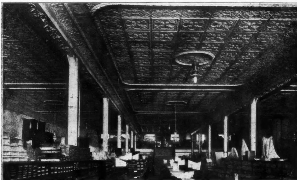
their slight increase in cost over lath and plaster. Closely joined, or interlocked, so as to make them easy and economical to install, they present an almost air-tight surface and being incombustible, they tend to greatly protect floors and woodwork in cases of fire, and have many times, by preventing the spread of flames until the arrival of the fire department, saved buildings from destruction. Being of
