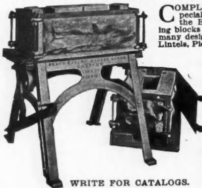
COMPLETE in every detail. Especially adapted to the use of the Block manufacturer. Making blocks in all widths, lengths and many designs, including Sills, Lintels, Pier Blocks etc. PRICE \$100
