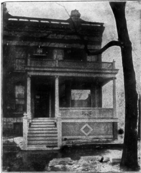
will invariably regret it within a short time, as it is almost impossible for a porch column, which is exposed to all the various changing conditions of the weather to stand, without coming apart, unless it is staved and built up with a good lock joint.
