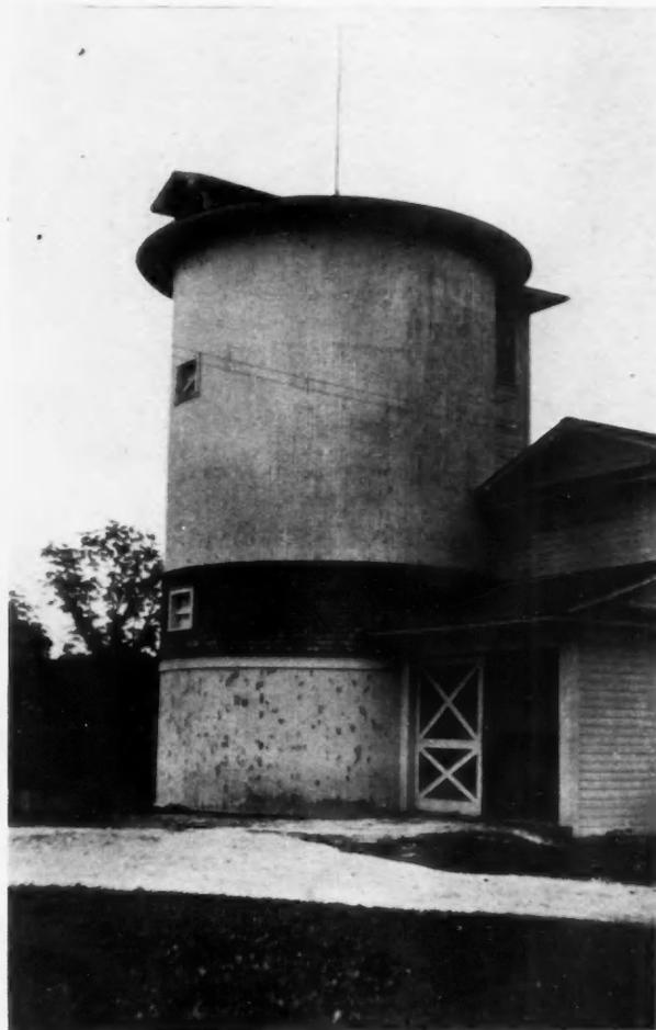
prevent this pressure from bulging out the walls the silo has been built in the shape of a cylinder. The sheathing boards on the inside and outside surface of
