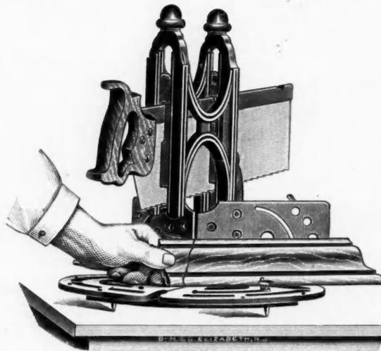
idea, which are fastened to the backs (see illustration) boards fourteen inches wide may be sawed with a twenty-four by four inch back saw to fit any angle, not only mitering the edge, but also the face of the board, making these attachments indispensable when cutting bases for pedestals and columns, base and other finishings around square and octagon corners. The machine can be knocked down in less than a minute's time, so that it will only take space in chest six by sixteen
