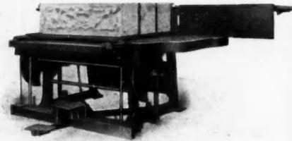
**No. 3.** 3 blocks moulded 8x32 inches. Mould box open ready to off bear blocks. See pallets and divisions. Cores are withdrawn by stepping on compound lever.
