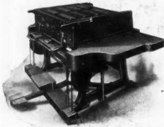
**No. 4.** Set to mould 4-6x32 inches. Machine is closed. Cores are raised and locked automatically by stepping on lever.
