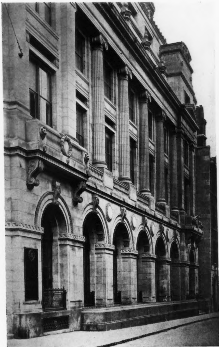
P. & O. BANKING CORPORATION, ST. MARY AXE, E.C. COLLCUTT & HAMP, ARCHITECTS.
