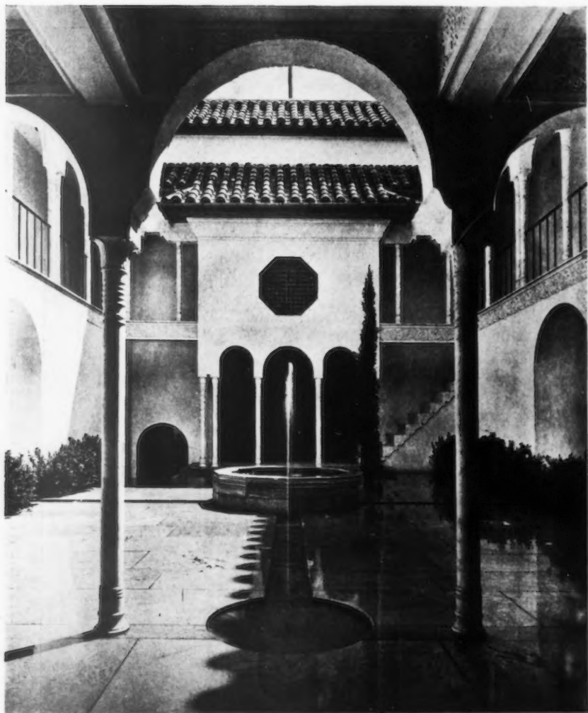
PATIO LOOKING SOUTH, PORT LYMFNE, NEAR FOLKESTONE.
