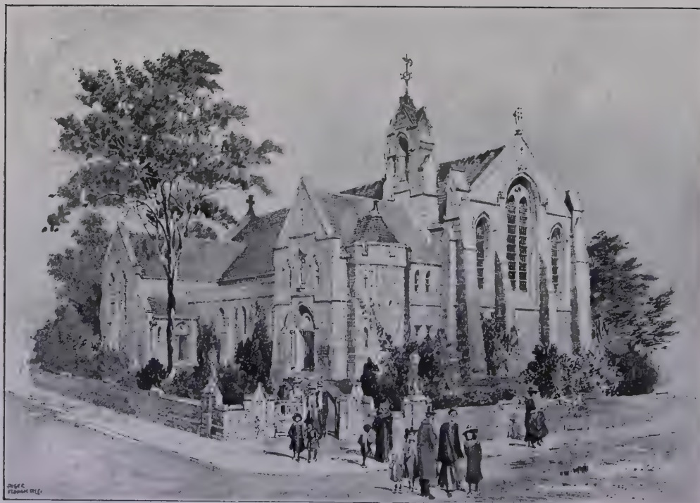
Village Church, Blackridge, J. GRAHAM FAIRLEY, Architect.
