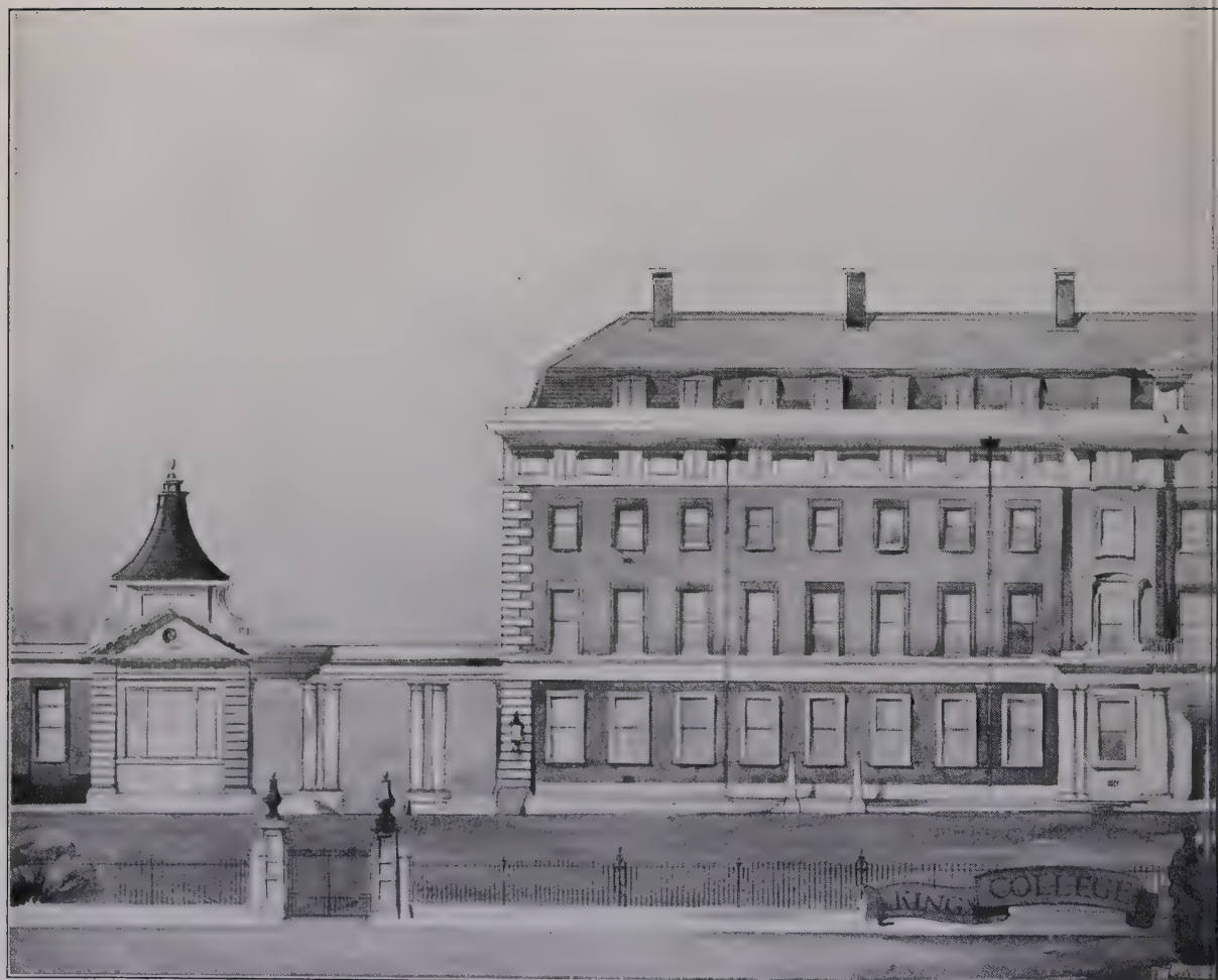
King's College Hospital, General Contractors: L. Hennebique Ferro-Concrete: L. G. Mouchel and Partners Sanitary Work and Drainage: Matthews
