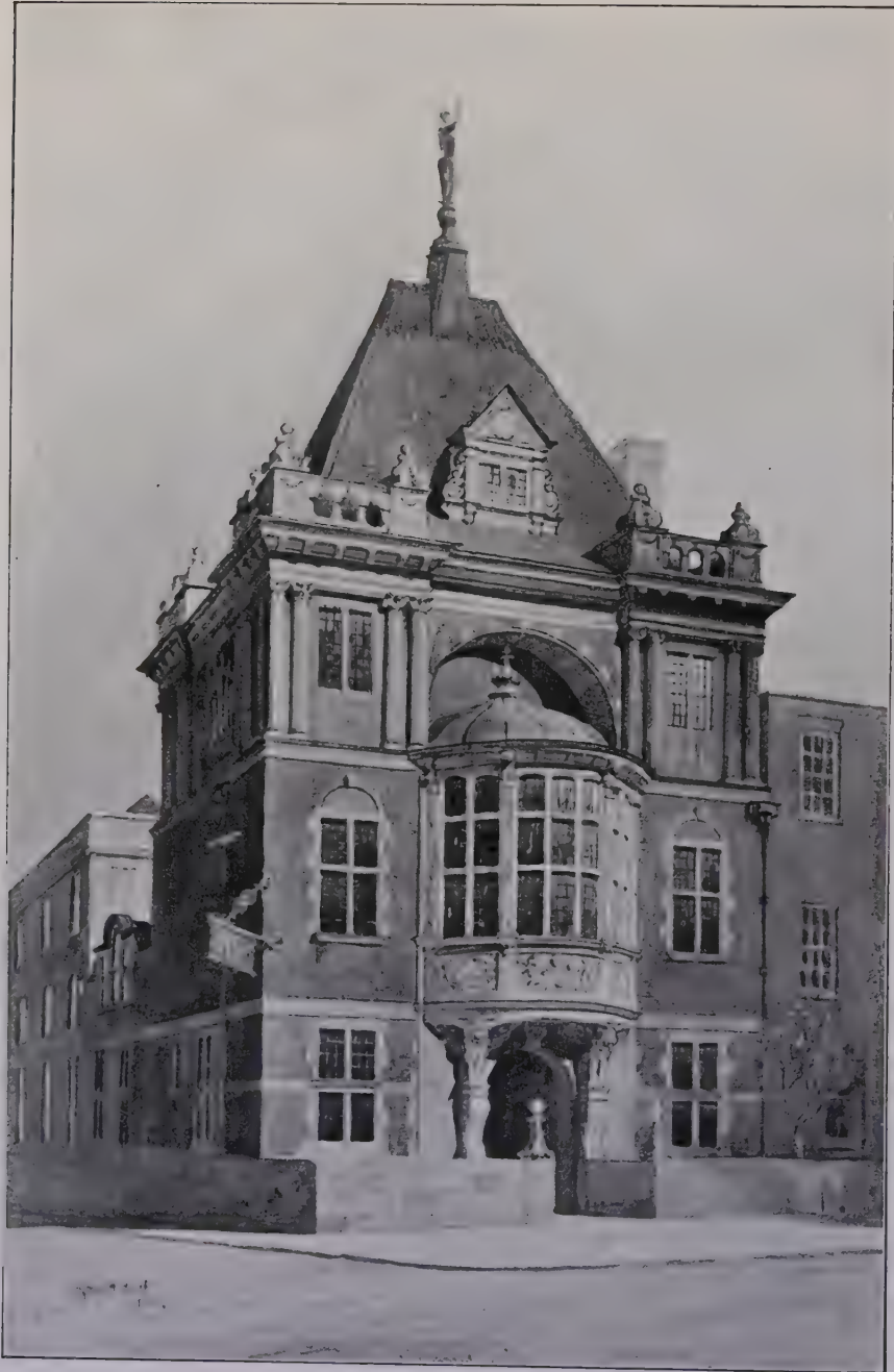
Office Building, London, HART AND WATERHOUSE, Architects.
