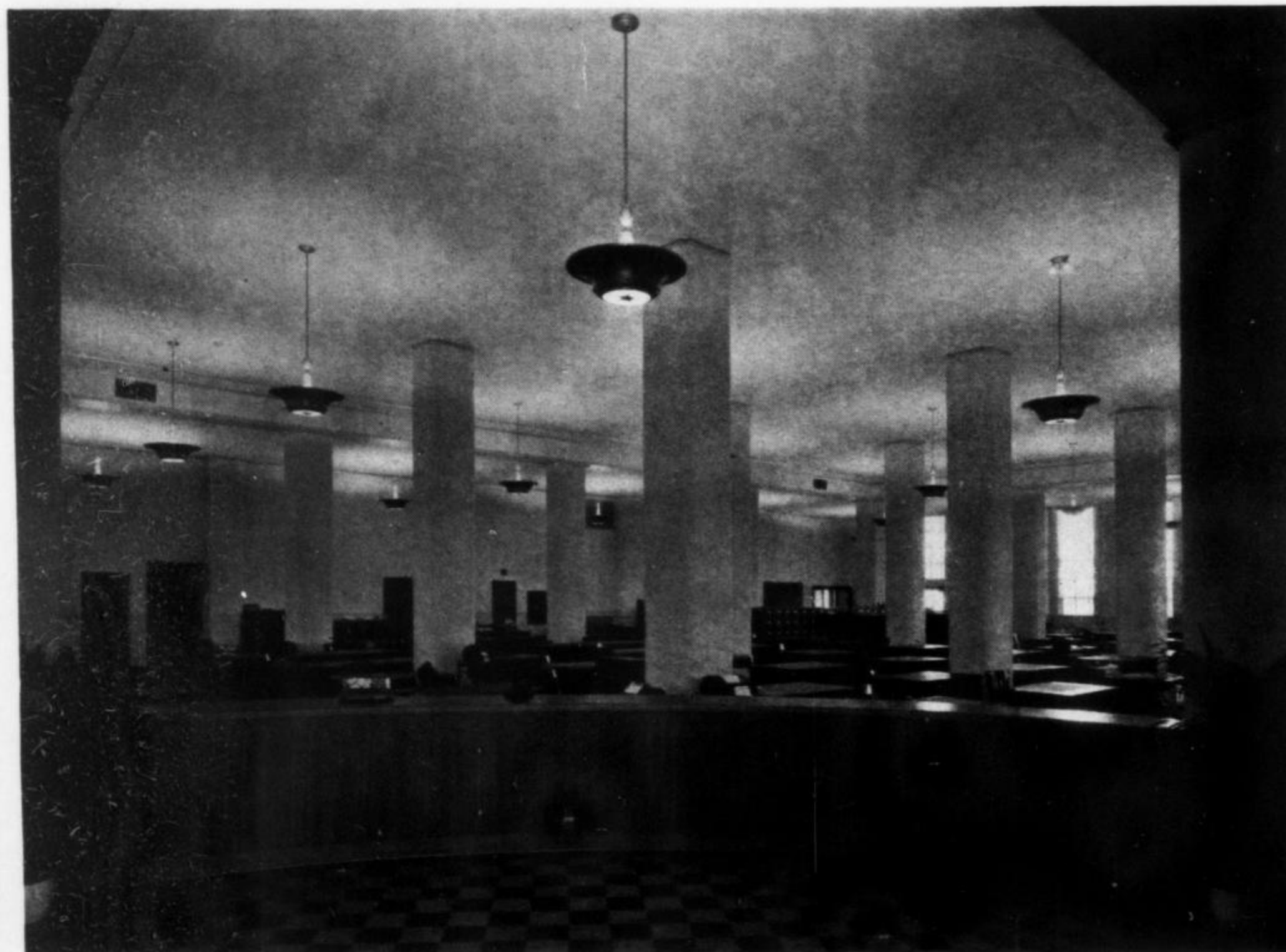
Part of main floor showing acoustical treatment with the use of Acoustite
