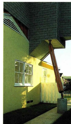
Buttress supporting second-story addition
