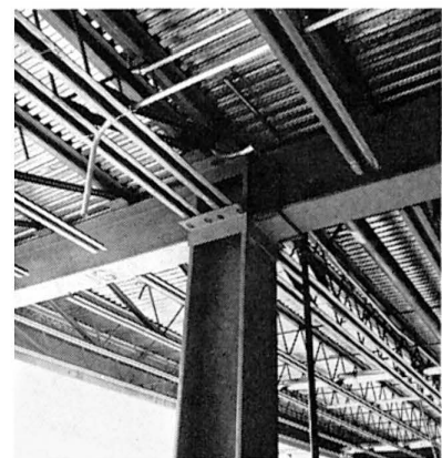
Steel joists allow pipe, conduit, and ductwork to be run in any direction.
