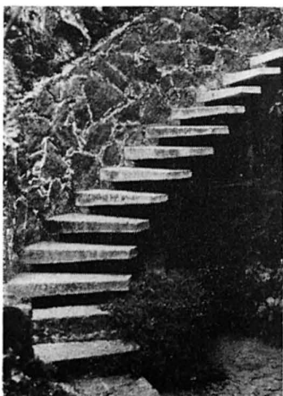
Above: east wall of bedroom terrace of O'Gorman house. Below: (left) concrete slab stairway cantilevered out from lava rock; (right) approach to the house with mosaic facade of Aztec symbols.
