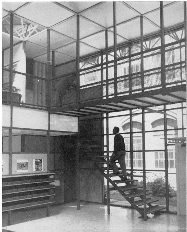
View of stairway and interior bridge One ceiling panel has been left out so that visitors can see into flux plenum
