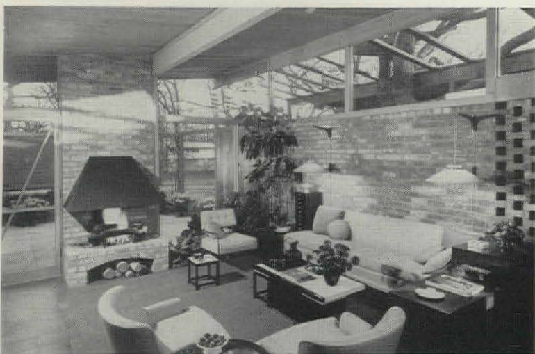
Cavity wall at right ends in brick lacework separating living area from entrance hall. Simple post-and-beam construction permits large unbroken areas of glass.
