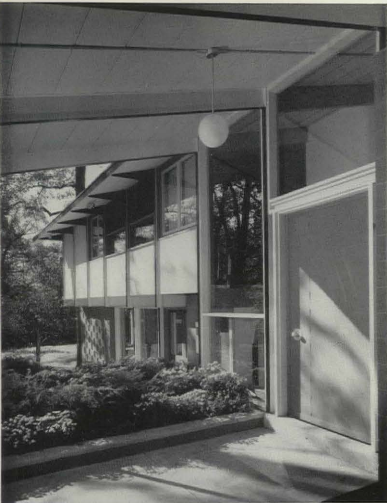
Entrance lies beneath an extension of the main roof over house and carport. Lower wall is built of interlocking concrete block, with alternate blocks turned edgewise for pattern.
