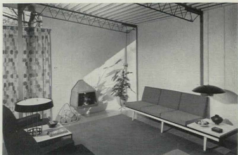
The house's structure—lightweight steel bar joists and steel roof decking—left exposed inside to give the space above eye level a pleasant texture and pattern.
