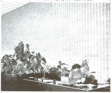
The C.B.S. "Eye" in concrete tile designed by Pereira & Luckman, architects, and custom fabricated by
