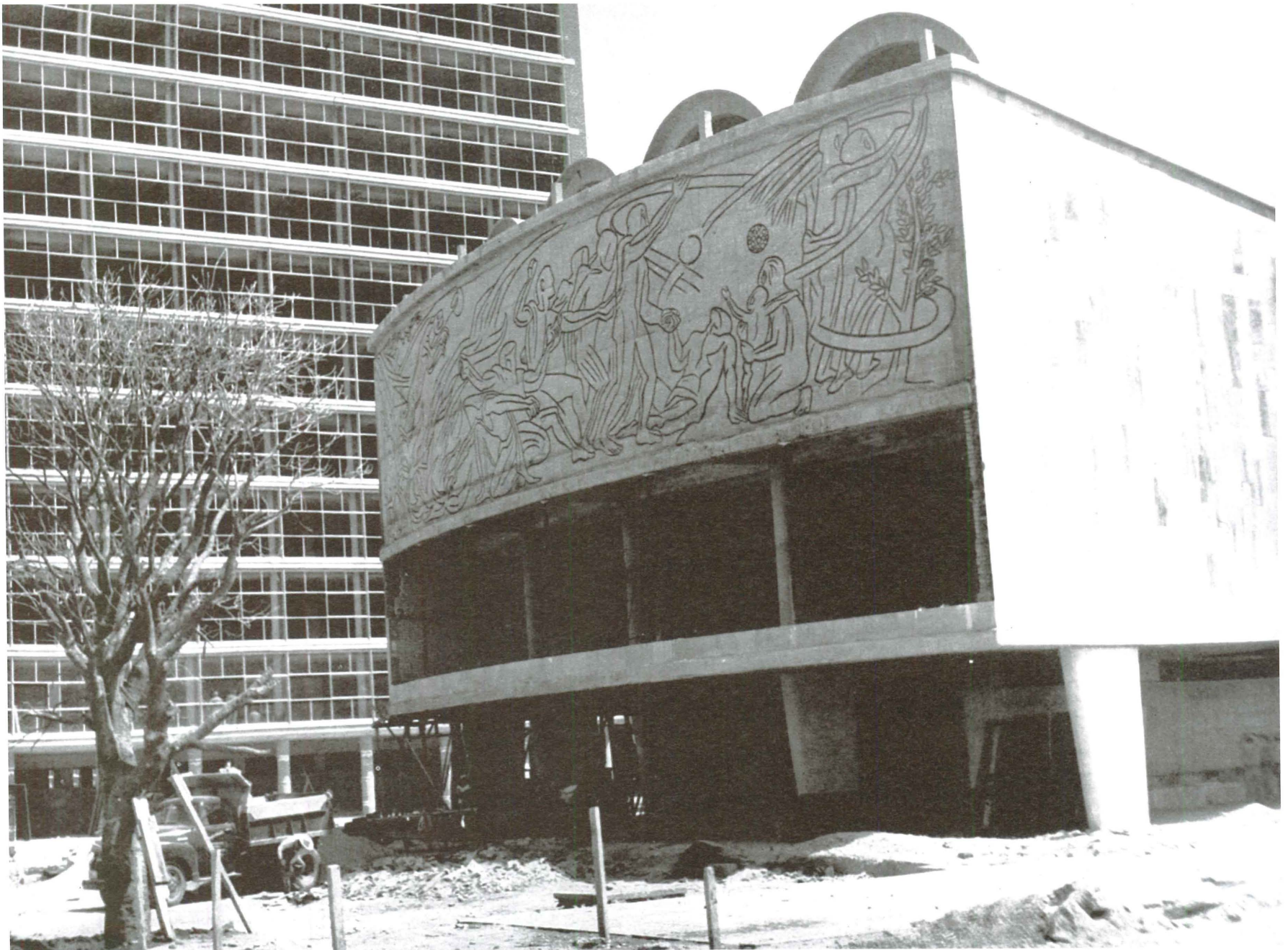
Below: Science Auditorium, with glazed side of Science Tower in background. The construction of the roof of the auditorium makes no interior obstructing support necessary. Mural on the south facade is by Chavez Morado and depicts man's conquest of an energy greater than fire. The travertine marble used on the exterior walls was quarried in the State of Durango.
