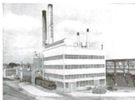
Attractive and economical use of alternate bands of glass and Cemesto for power plant at Good-year Tire & Rubber Co., Jackson, Mich.
