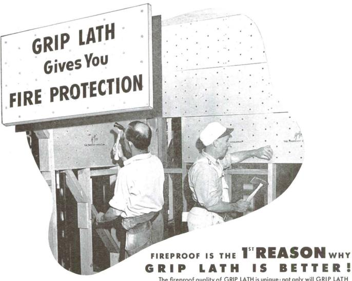
The fireproof quality of GRIP LATH is unique; not only will GRIP LATH not burn or support combustion, but high temperatures cannot pass through it. The protection given by GRIP LATH and Gypsum Plaster safe-guards wood against fire. Fireproof GRIP LATH builds safer homes.
