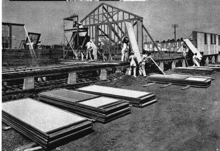
Modulok Cemesto Wall Units go easily into position in constructing the Naval Hospital at Corona, California.
