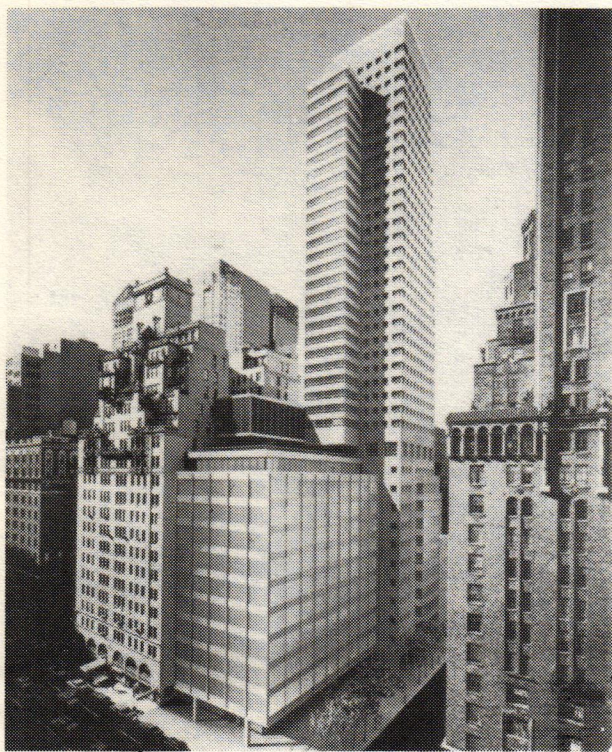
500 Park Tower montage (photo: Wolfgang Hoyt, Esto)
