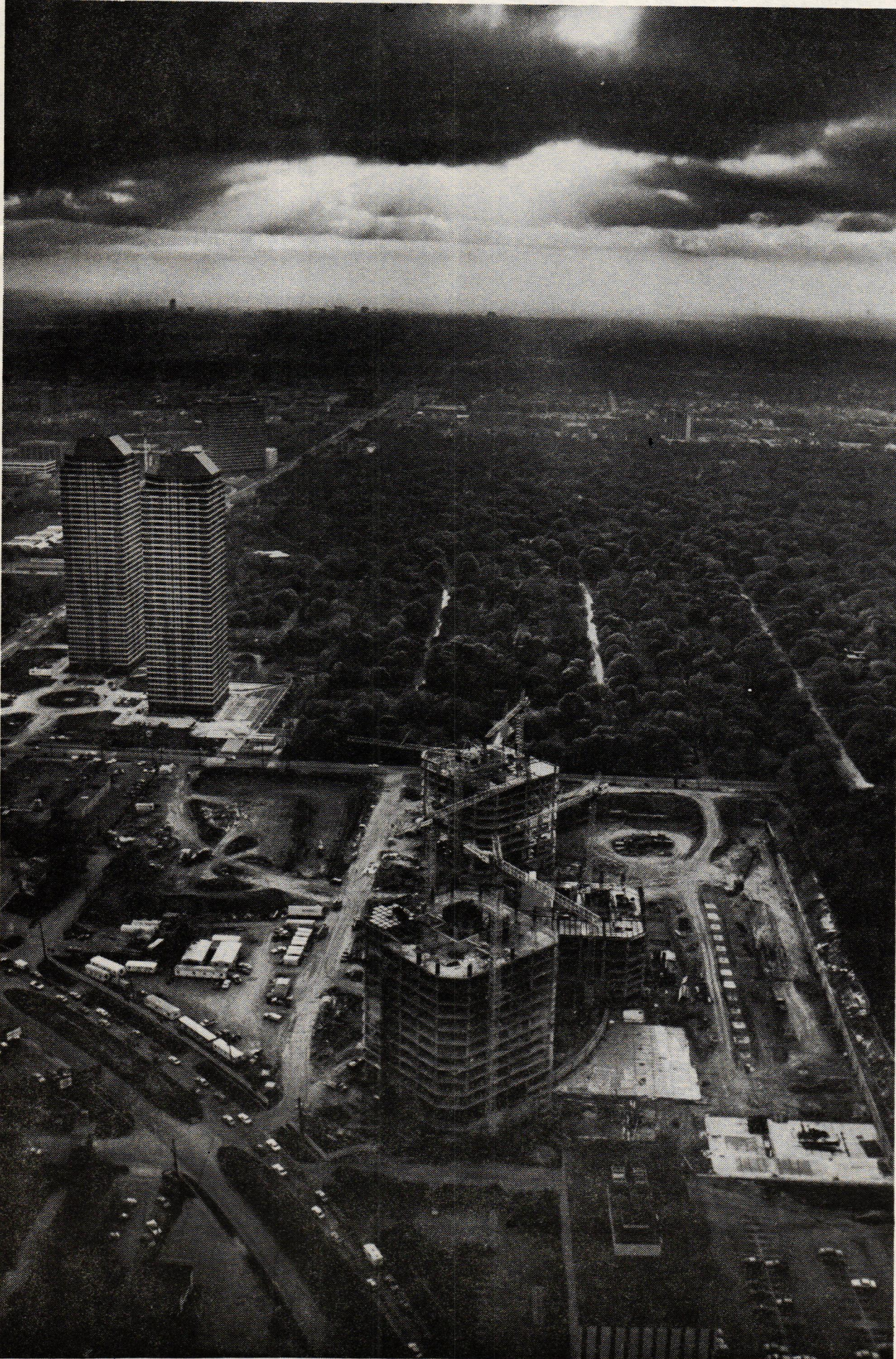
Aerial view of Four Oaks Place (front) and Four-Leaf Towers (back) (courtesy Cesar Pelli & Associates)
