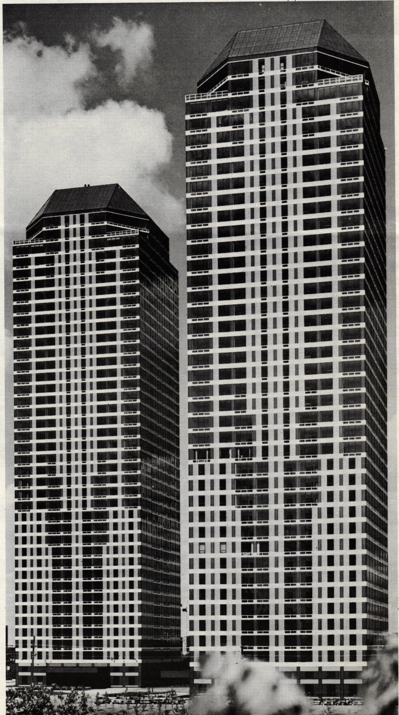
Four-Leaf Towers, Houston (1982); Cesar Pelli & Associates (photo: Balthazar Korab)
