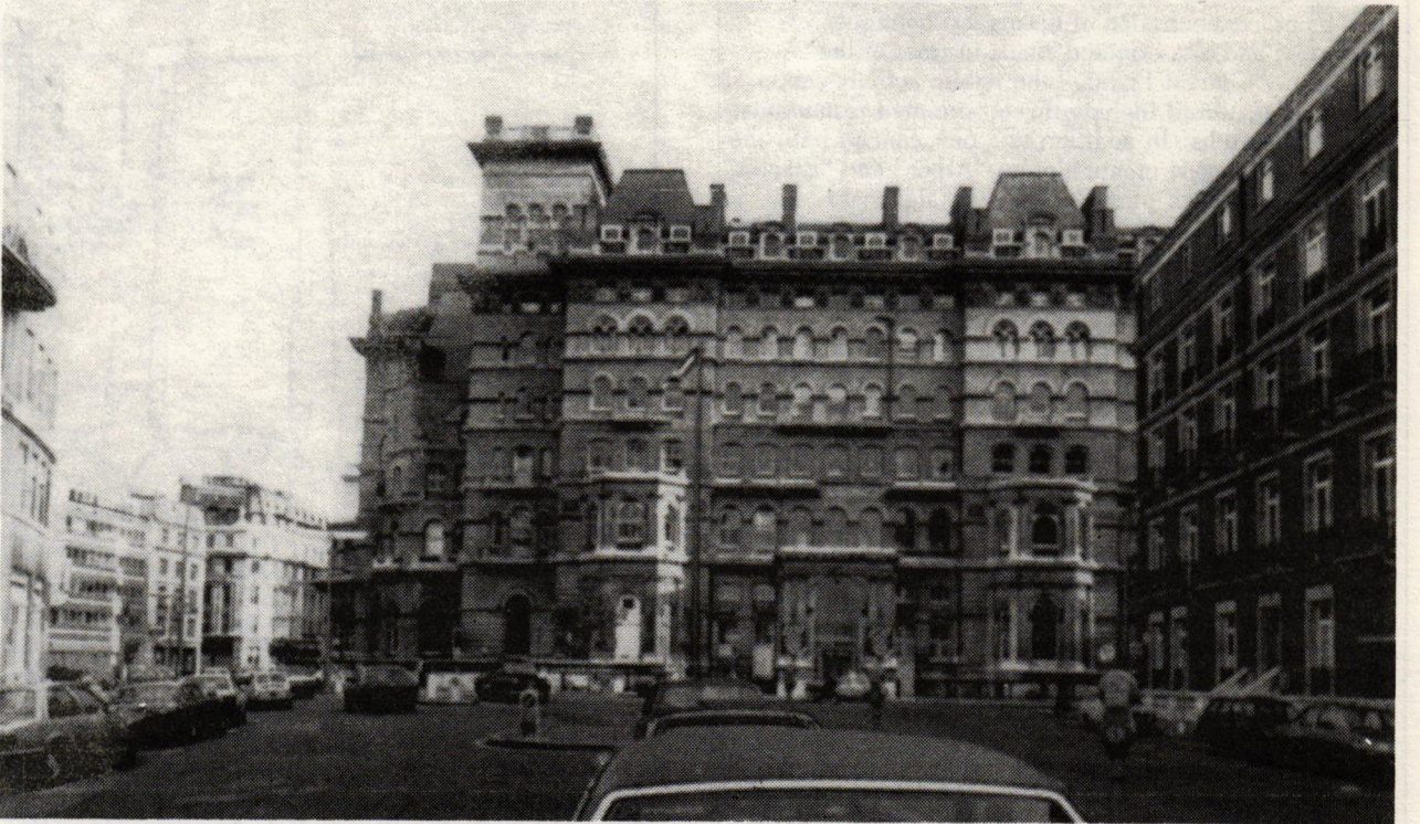
Langham Hotel, Langham Place, London (1864); John Giles and John Murray (photo: Steven Groak)
