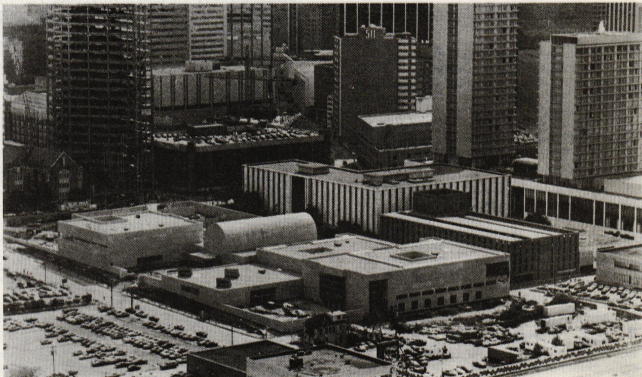
Dallas Museum of Fine Arts; Edward Larrabee Barnes. Construction shot at entrance (photo: Dan Barsotti)
