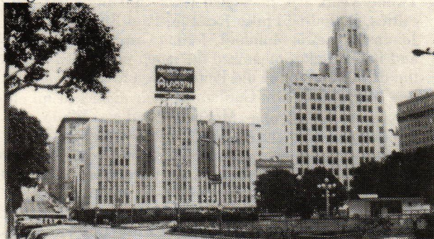
Today, as "updated" in 1938 (photo: Robert Coombs) the garage. Above the portals are large tile murals depicting scenes of progress. The soffits of the portals are worked with interlacing geometric Moorish tile patterns. Large bronze lanterns in a streamlined Spanish Baroque style complete this aspect of the design. This approach is countered by other Egyptian- and Greek-inspired Deco elements, such as the magnificent bronze gates of the portals.
