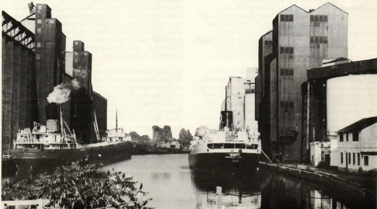
View of the Buffalo River and grain elevators from the Ohio Street Bridge, Buffalo, N.Y. (photos: Patricia Layman Bazelon)
