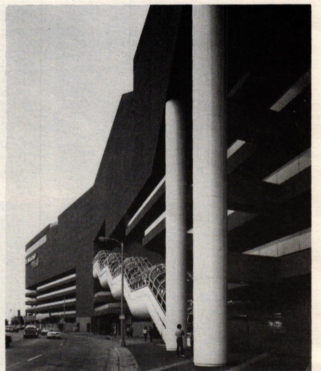
Exposed escalators along Beverly Blvd. (photos: Bielenberg)
