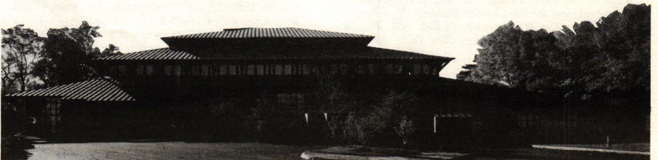
View toward lecture hall (south elevation).
