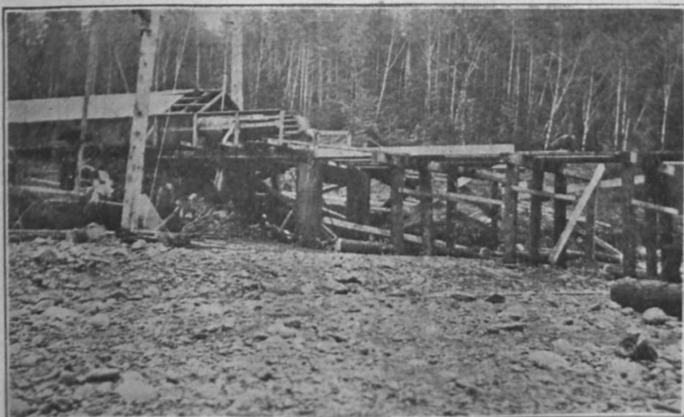
Repairing Break, Cedar River Pipe Line Near Lansberg, November 20, 1911
