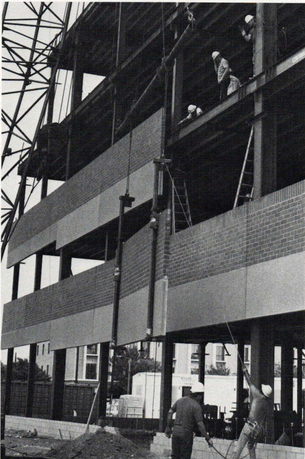
Prefabricated brick panels are lifted into place and connected to the frame of the building.
