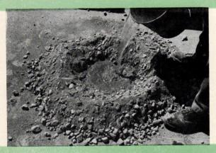
Gravel is thoroughly mixed with cement and sand until there are no streaks of brown or gray. A depression is formed in the middle of the pile and the correct amount of water poured in. A ten-quart pail, marked off inside to indicate quarts and gallons, makes measurement of water easy.
