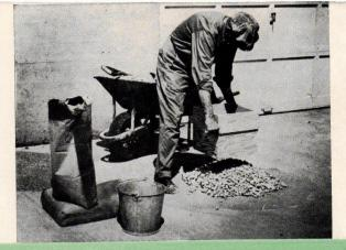
A bottomless box, constructed one foot square to hold 1 cu. ft. of material, simplifies measurement of sand and gravel. A measured amount of sand is spread on a flat surface. The proper amount of cement is added, and the two mixed together. A measured amount of gravel is then placed on top of pile.
