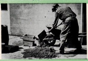
After water is added, mixing is resumed until all ingredients are thoroughly and uniformly combined. Every piece of stone should be completely coated with the mixed mortar. A good concrete mix for around-the-home jobs looks like one below after the surface has been troweled with a shovel. The mix is fairly stiff and not "mushy." Concrete should be placed in the forms within 30 minutes after mixing.
