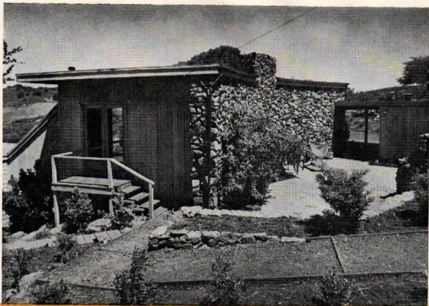
The patio area always gets the morning sun. Rock in the wall is native stone. The door at the left leads directly to the living room.
