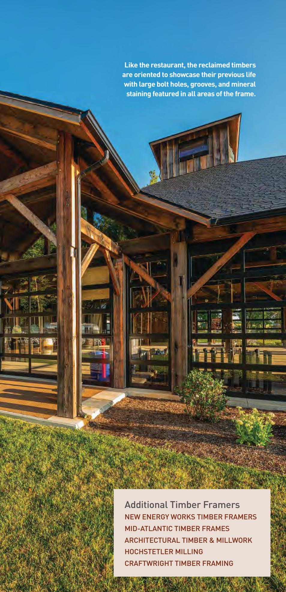
Like the restaurant, the reclaimed timbers are oriented to showcase their previous life with large bolt holes, grooves, and mineral staining featured in all areas of the frame.
