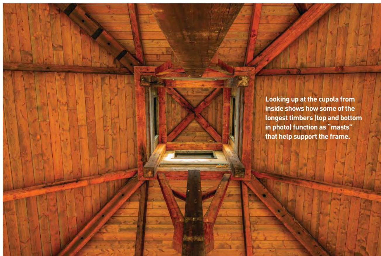
Looking up at the cupola from inside shows how some of the longest timbers (top and bottom in photo) function as "masts" that help support the frame.
