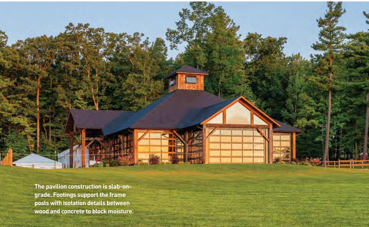
The pavilion construction is slab-on-grade. Footings support the frame posts with isolation details between wood and concrete to block moisture.
