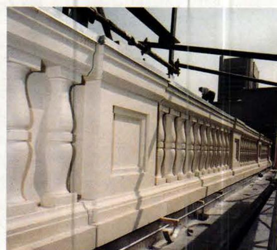
Above right: A spindly 1914 balustrade, made of cast iron or terra cotta, had failed and been removed by the 1950s, and a 1980s replacement was cobbled together from turned posts and plywood. Beyer Blinder Belle's GFRC substitute, with wider balusters than the original, helps conceal a rooftop recording studio added in the 1980s. *Photo: Bernstein Associates*
