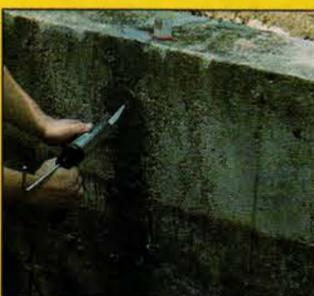
**AboJet** series for structural crack-injection
