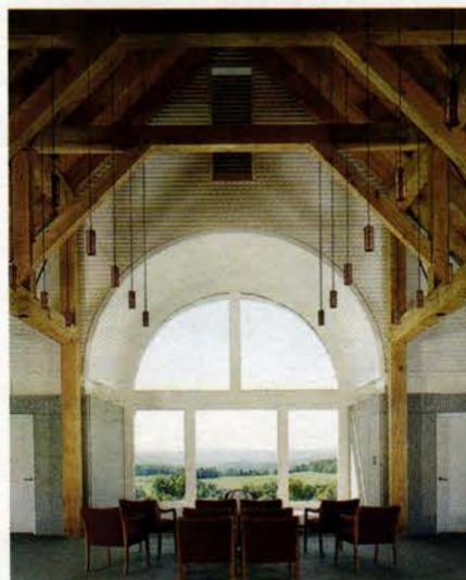
The Vermont Veterans Memorial Chapel in Randolph, VT, was built by Vermont Timber Works using natural and glue-laminated timbers and traditional mortise-and-tenon joinery.
