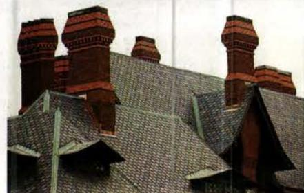
Kronenberger & Sons' restoration of the exterior of the Mark Twain House in Hartford, CT, included masonry raking and repointing, as well as replacing the chimneys following a corbelling design found in historical photos.
