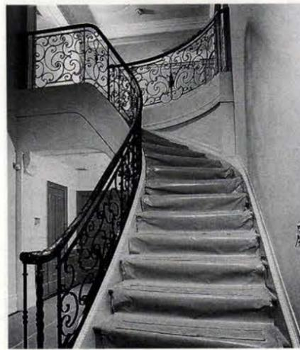
This French Provençal stair rail, manufactured by John F. Graney Metal Design, measures 28 ft. long.
