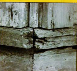
Consolidation & rebuilding of rotted windowsill with LiquidWood & WoodEpoxy .
