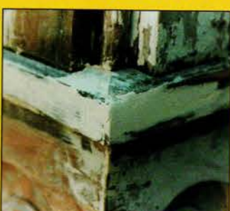
Consolidation & rebuilding of rotted windowsill with LiquidWood & WoodEpoxy .
