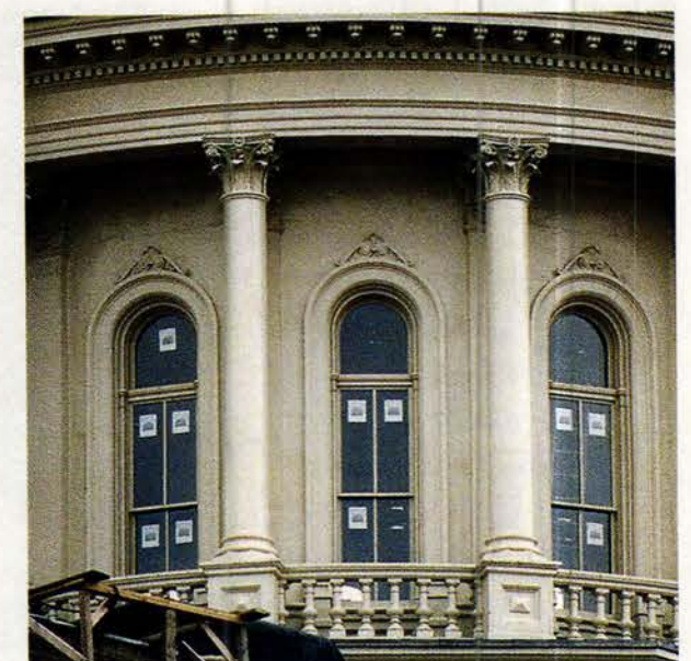
These mahogany windows with insulated glass were custom manufactured by Adams Architectural Wood Products . Write in No. 1265
