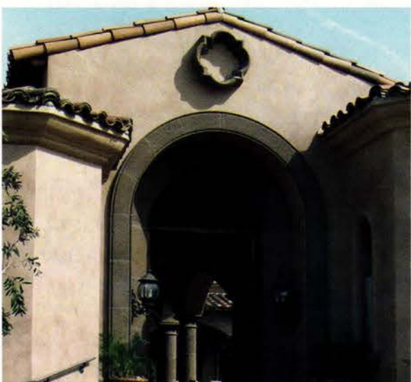
Seawright Custom Precast fabricated the arched trim, quatrefoils, window sills, wall caps and stackable columns for this building in La Quinta, CA. Write in No. 1154
