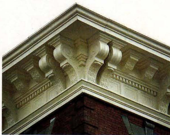
Architectural Fiberglass Corp. replicated the original 61-in.-tall cornice with a 30-in. projection for this landmark building in the Bronx, NY. Write in No. 6400
