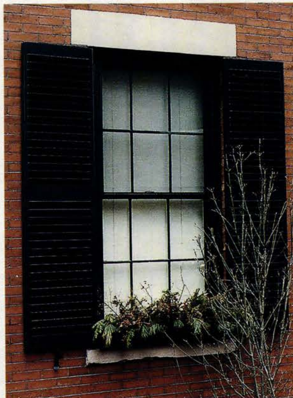
Beech River Mill manufactured these 1 3/4-in.-thick shutters that feature a 2 3/4-in.-wide fixed slat with scalloped corners projecting beyond the face of the frame-stock. Write in No. 4110
