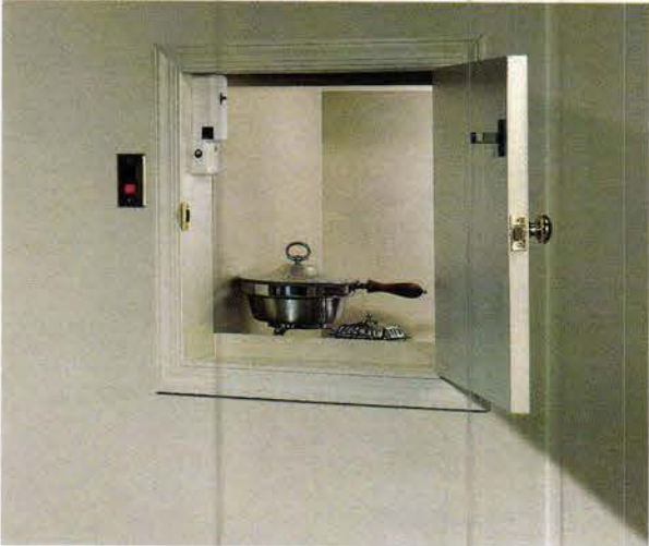
Inclinator's Homewaiter has a travel distance of 35 ft. and opens on multiple sides.
