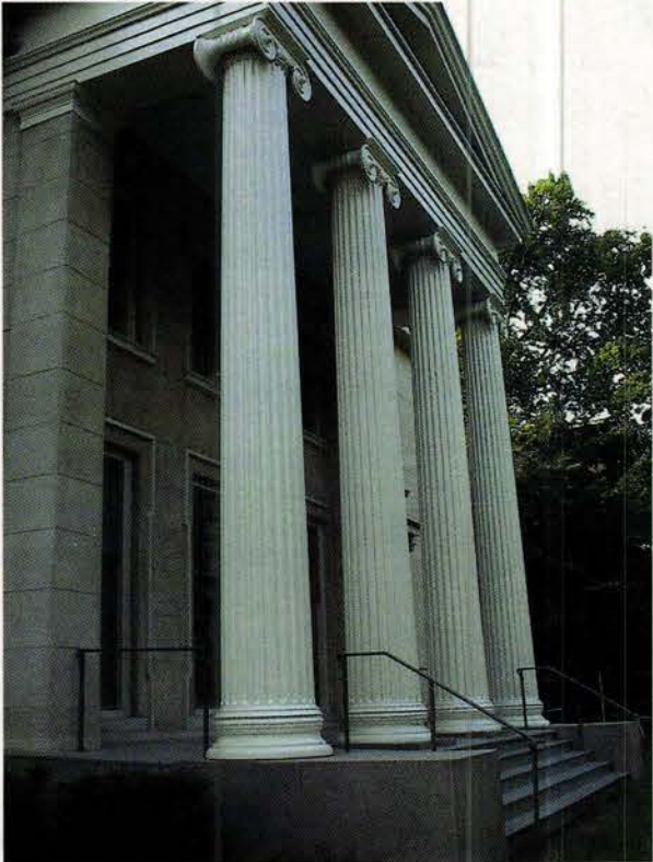
Fagan Design & Fabrication replicated this 30-in.-dia. x 20-ft.-tall fluted column (foreground) to match the existing columns. Write in No. 8210
