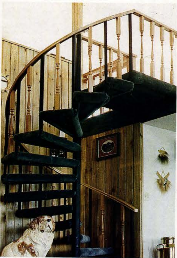
Fabricated by Goddard Spiral Stairs, this metal and wood staircase features center balusters of oak and solid-wood handrails. Write in No. 4780
