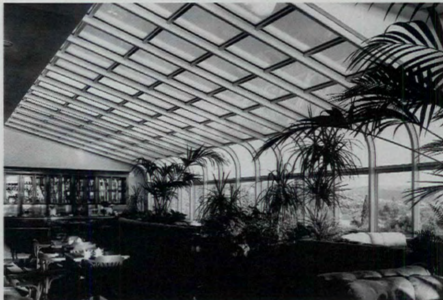
FOUR SEASONS SUNROOMS' System 5 line of commercial sunrooms and enclosures features an all-aluminum structure and curved-eave option, as seen here in the firm's work on the cafe and bar of the Grand Hotel Emona in Slovenia. Write in No. 910
