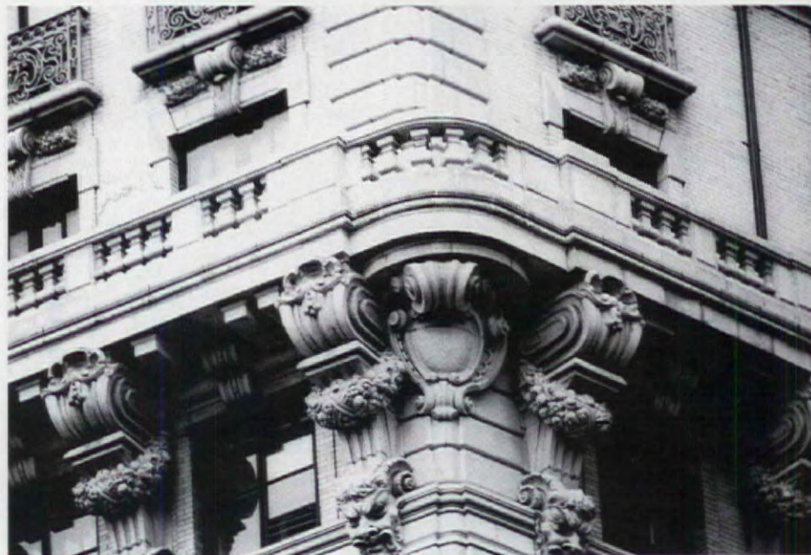
TOWNE HOUSE RESTORATIONS fabricated these balustrades in cast stone and GFR for the restoration of the Ansonia Hotel in New York City. Write in No. 545
