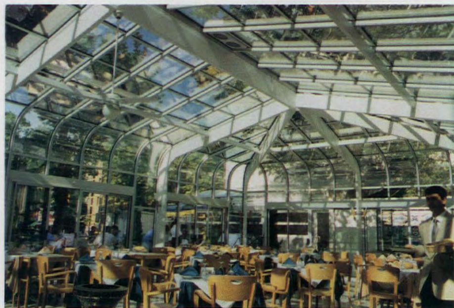
The main steel substructure of the addition, easier to see in this interior view, supports the slimmer lines of the structure and permits patrons to enjoy a open-air feeling.
