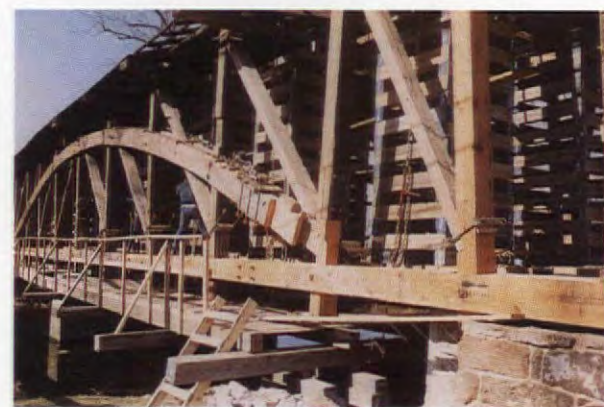
For the restoration of the Utica Mill covered bridge near Thurmont, Md., Dean Fitzgerald Heavy Timber Construction lifted the entire 101-ft. span, suspended with about 40 tons of cribbing, in order to replace 30,000 board ft. of timber, including 10-12,000 board ft. of the Burr truss, with solid oak and yellow pine. The bridge dates from around 1843 and was originally built over the Monocacy River. It was washed out in the Johnstown Flood of 1889 and rebuilt, in a truncated form, at its present location in 1891.
