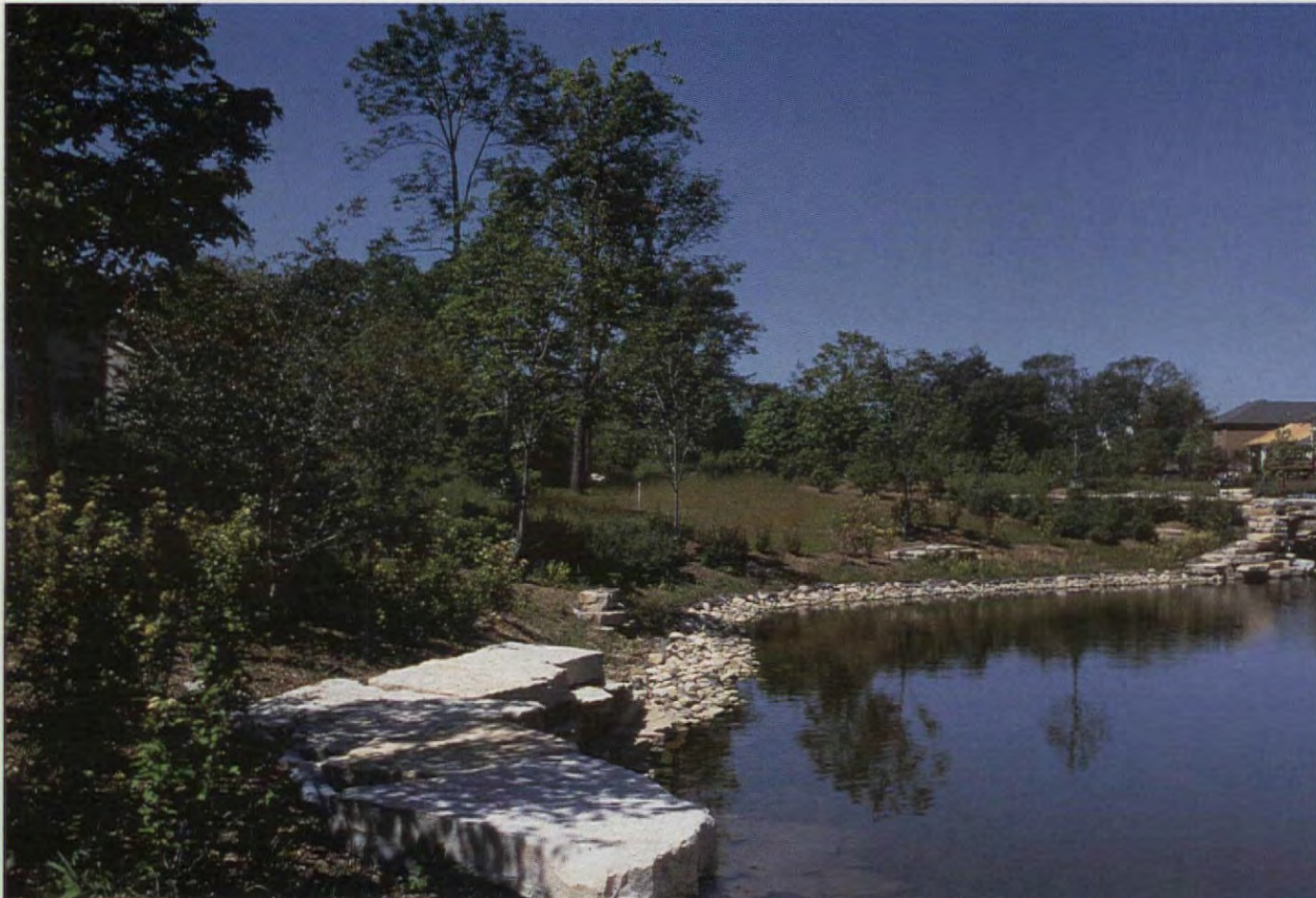
Edged in limestone and enhanced with perennials, this new storm-water-detention pond was added to provide detention required by the increased number of residents. (Photo: Bernard Jacobs - Jacobs/Ryan Associates)
