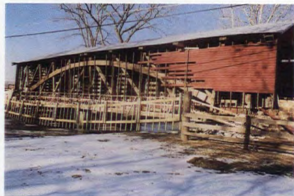
A major aspect of the project was the removal and refurbishment of the bridge's siding and shingle roof. Over 70 percent of the original siding was reused and an entirely new roof put in place.
