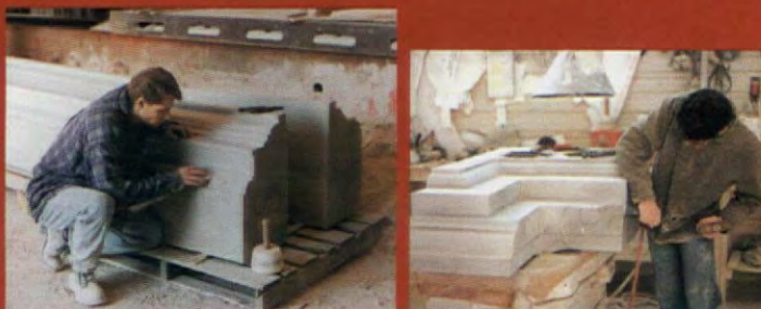
Stonecutters carving and finishing Scioto sandstone for restoration of the Filson Club
