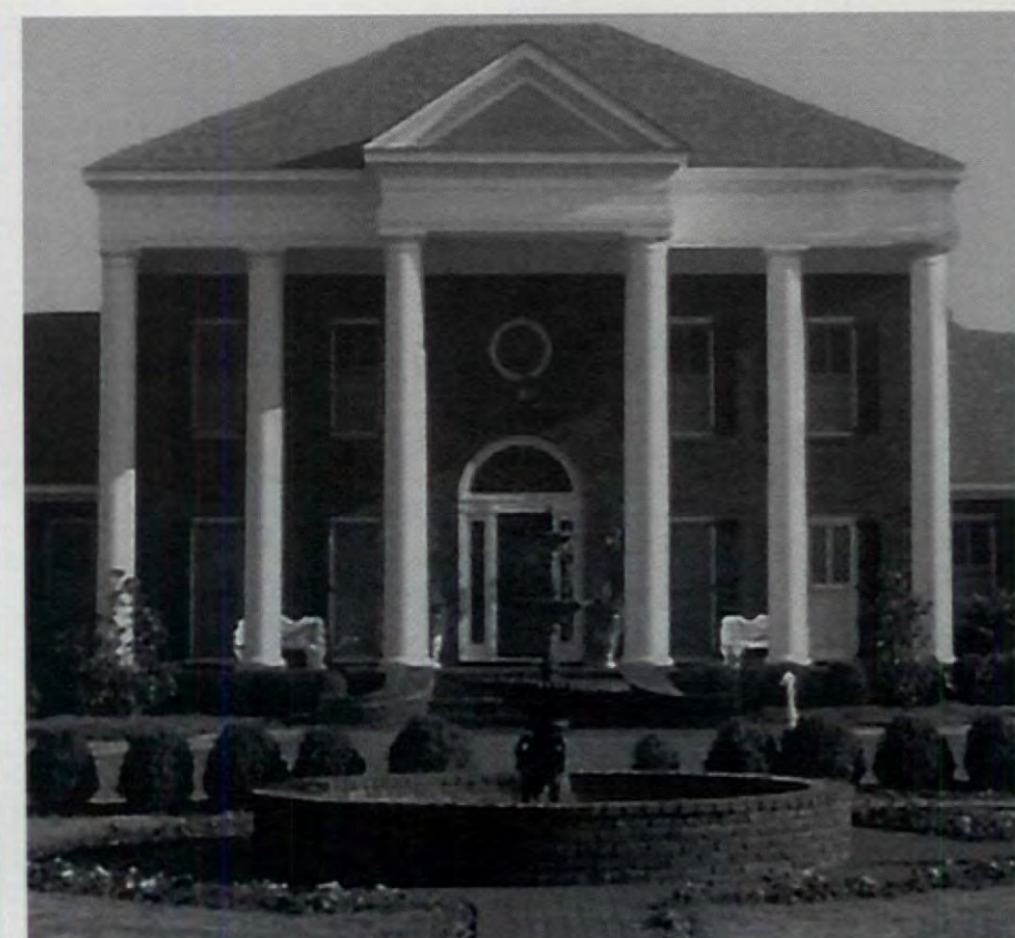
CAMMCO's columns, made of fiberglass-reinforced polymer, are available in a variety of standard sizes or, as pictured here, in custom lengths. Write in No. 2566
