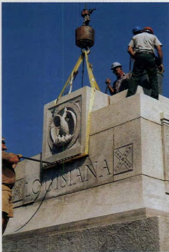
A crew dismantles the base of the Louisiana Monument in Vicksburg, Miss. Both the base and the column that sit upon it are Dorian Gray Granite, and both were severely damaged by lightning in May 1999. LAS provided technical supervision for the dismantling of the monument. Restoration is currently awaiting funding. (Photo: LAS)
