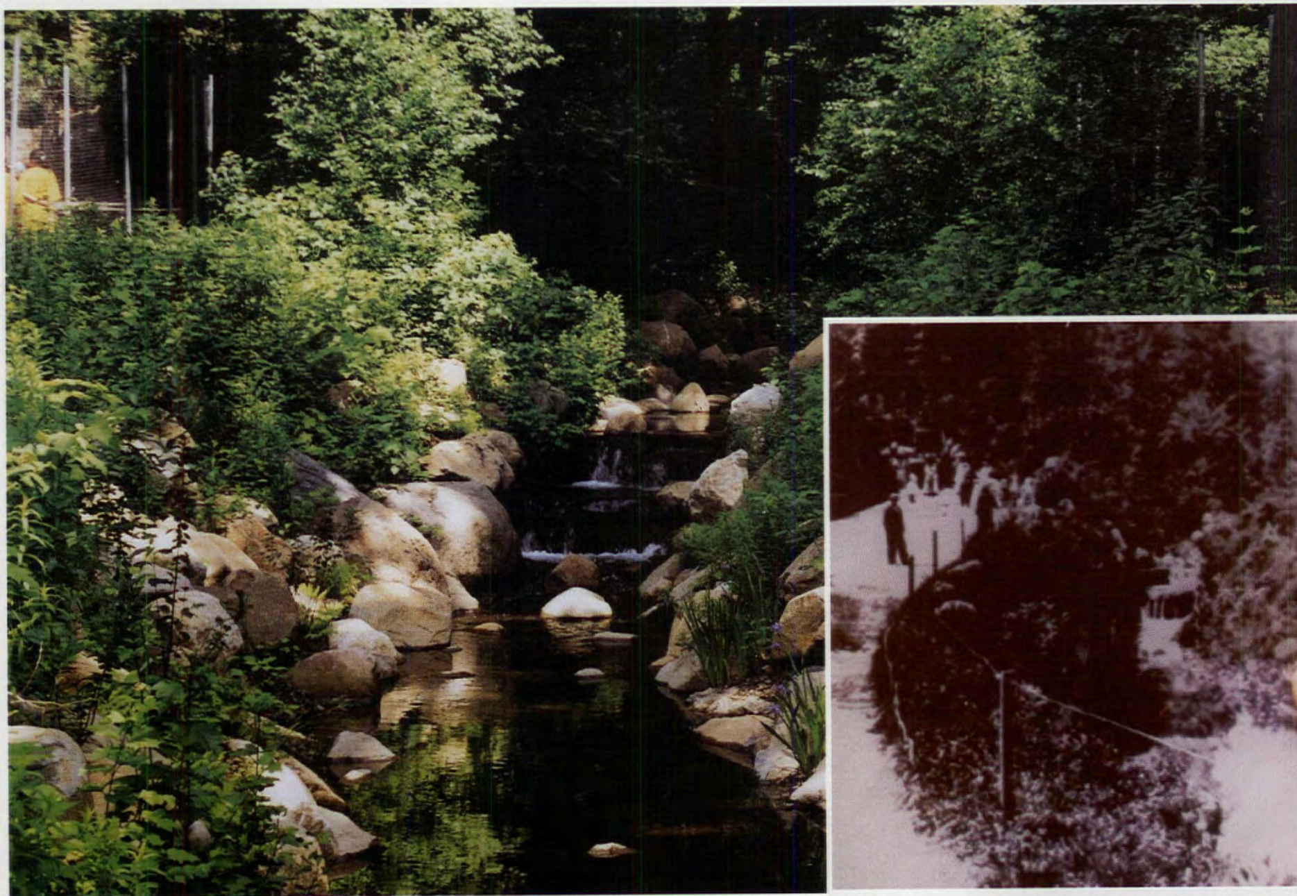
The historic photo (inset) revealed that the path here once curved in harmony with the water course, but had been straightened by a subsequent designer, and that there was once an important waterfall, since buried. The path was restored to its original gracefulness and the fall disburdened of sediment. The fall had been constructed such that water flowed into a hollow beneath the top stone, creating a reverberation audible from the carriage bridge from which the historic photo was taken.
