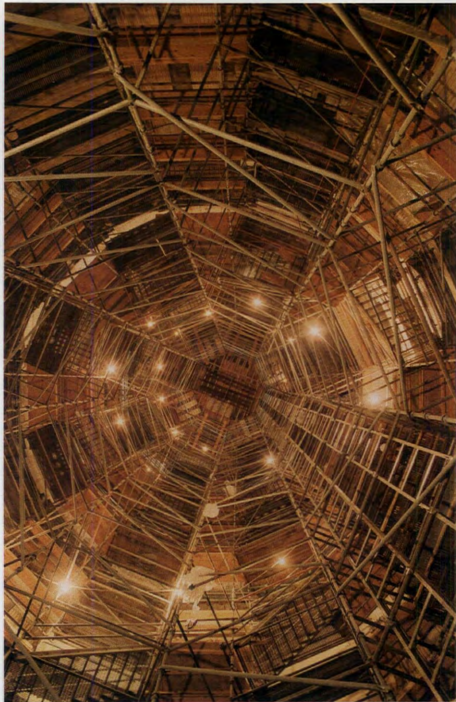
The same rotunda under scaffolding. At 168 feet the scaffolding itself is impressive. (Photo: Jonathan Hillyer/Atlanta)
