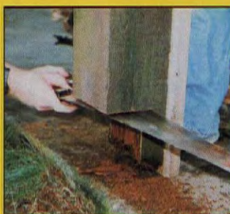
Rotted & infested base of a loadbearing column is completely sawed off & replaced with WoodEpoxy .
