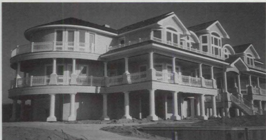
HB&G supplied 118 PermaCast, fiber-reinforced polymer columns for this building on Pine Island, N.C. Write in No. 580
