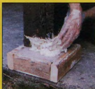
Rotted & infested base of a loadbearing column is completely sawed off & replaced with WoodEpoxy .
