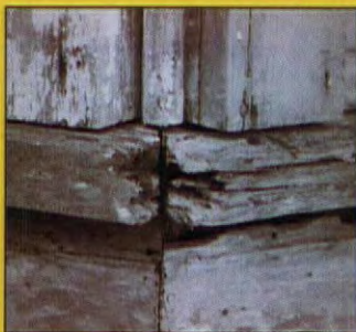
Consolidation & rebuilding of rotted windowsill with LiquidWood & WoodEpoxy .
