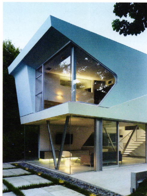
Alan-Voo Residence addition in Los Angeles by Neil Denari
