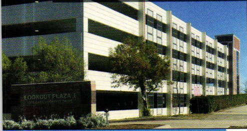
BEST PARKING STRUCTURE (Small) East Lookout Parking Garage
