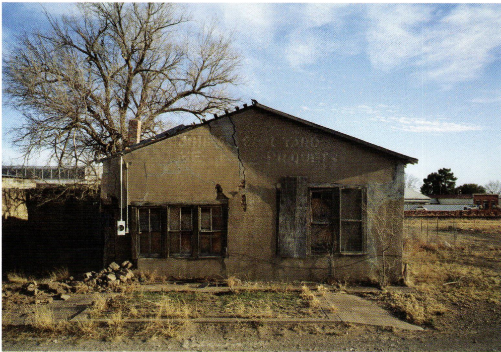
Ruined adobe building, Marfa.
