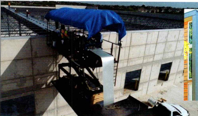
High Lift truck offers lap-free joints reducing costs and time.
